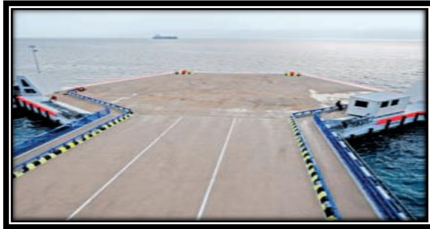
Figure (4): Triple-berth pontoon linkspan
